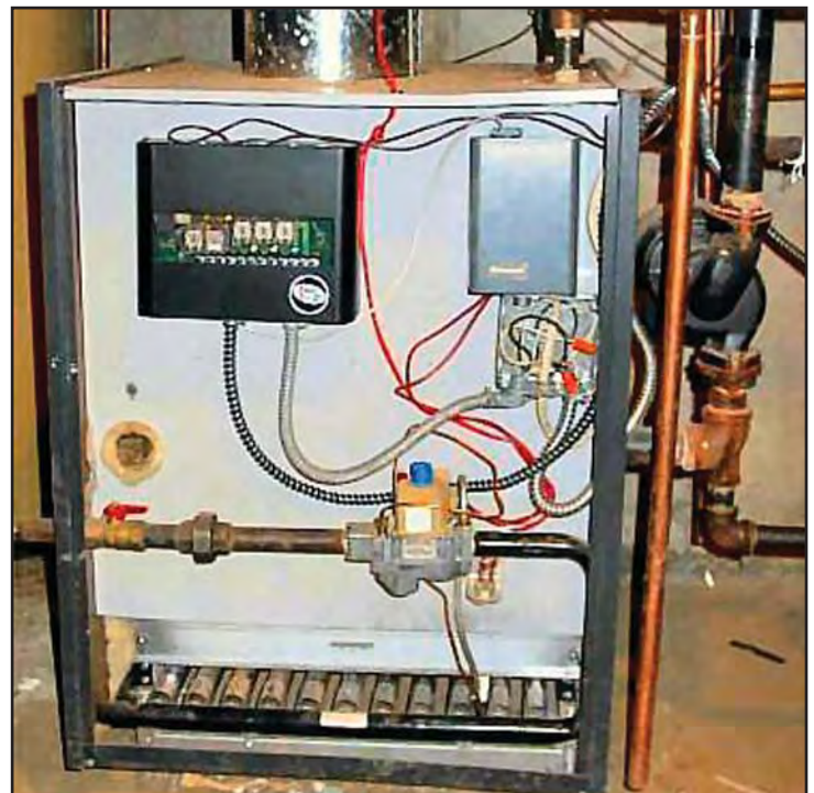
Figure 12.9. Gas-fired Boiler
