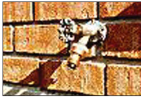
Figure 9.17. Hose Bib With Vacuum Breaker
