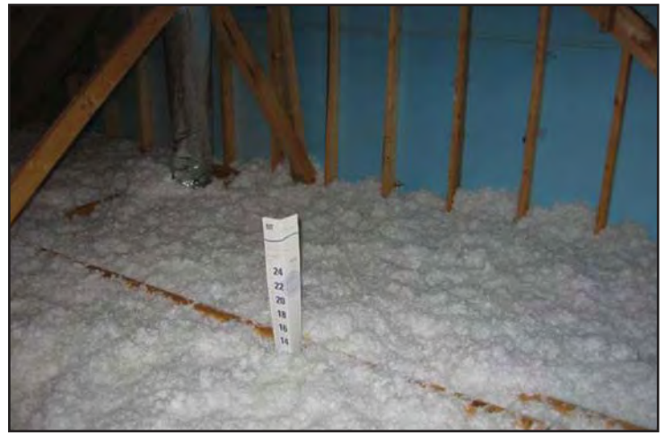
Figure 7.3. Depth of Attic Insulation
