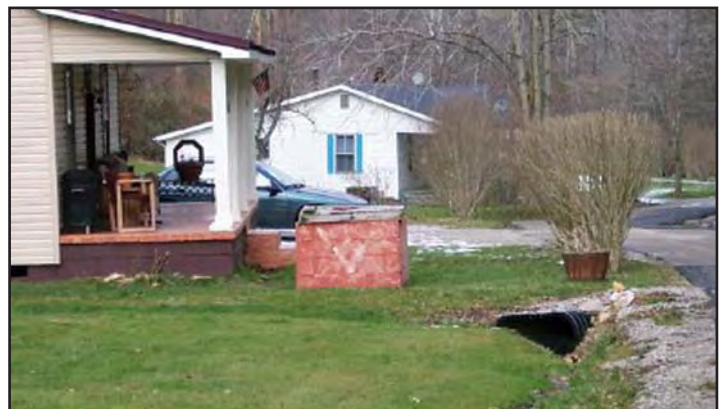
Figure 8.7. Typical Dug Well
